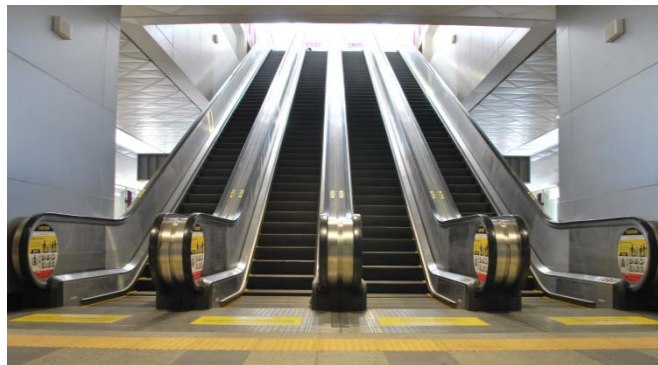
Escalators delivered to MRT Purple Line
